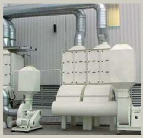
All our blastrooms are supplied with TDF (tru downflow) dust collectors to generate the blasting ventilation and or abrasive recovery airflow.
